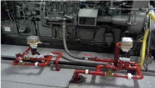
**Figure 8.** Erection of flow meter (after)
