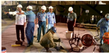
Gambar 2.13. Bottom Plate Automatic Welding
