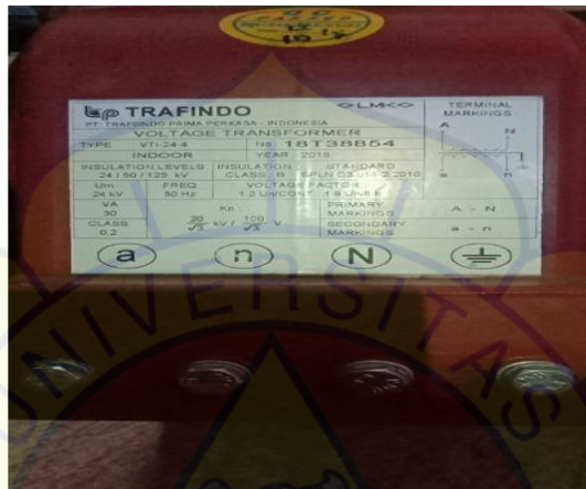
Gambar 2. 10 Voltage Transformator
