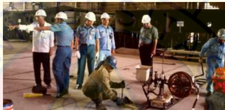
Gambar 2.13. Bottom Plate Automatic Welding
