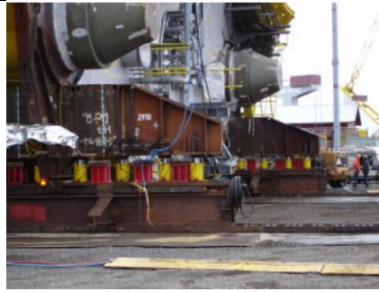
Gambar 2. 18 Skidding By Uniform Loading Using Hydraulic Cylinders
