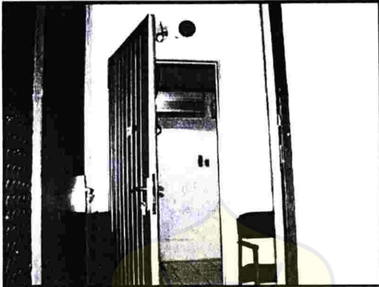
OVERVIEW SHELTER CONDITION
