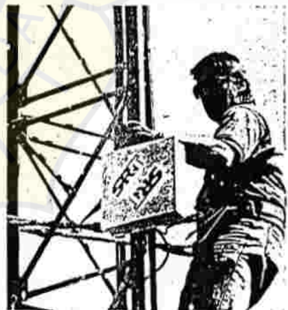
Antenna Integrated Module (AIM) of the 10.5GHz transceiver option
