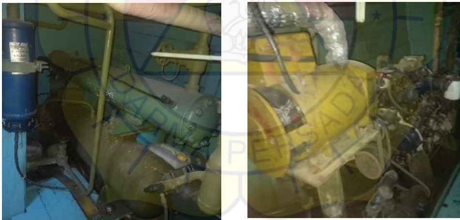
Gambar 2.21: RSW unit w/ Reciprocating compressor
