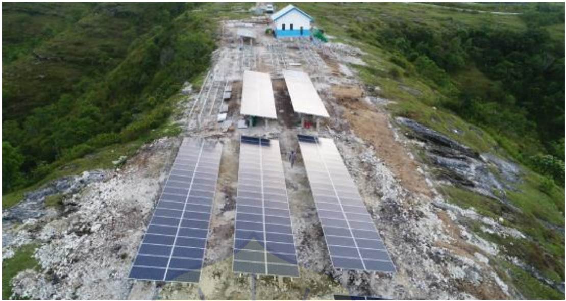
Gambar 2-4 PLTS Ground Mounted
