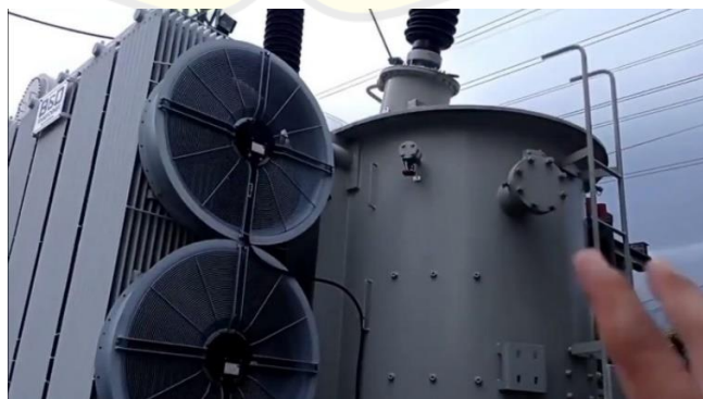
Gambar 2.9 Pendingin Transformator
